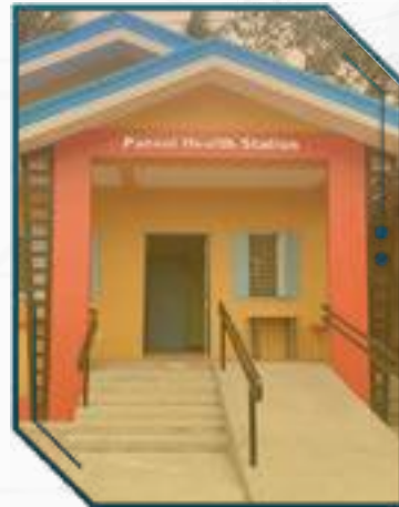
Pansol Health Station ■ ■
